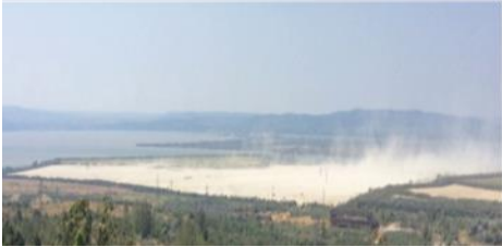
Figure 1 – A view of closed Moldomin mining company flotation tailing dump no.3, in windy conditions.
