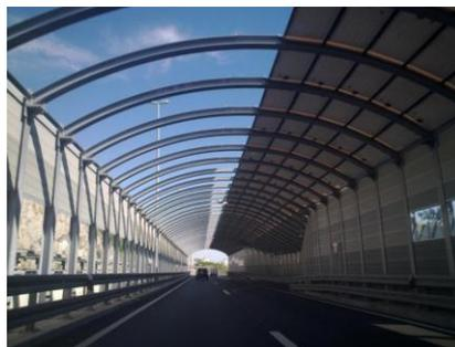
*Figure 6 – An example of how to reduce the level of noise on the road near the settlement, [7]*
